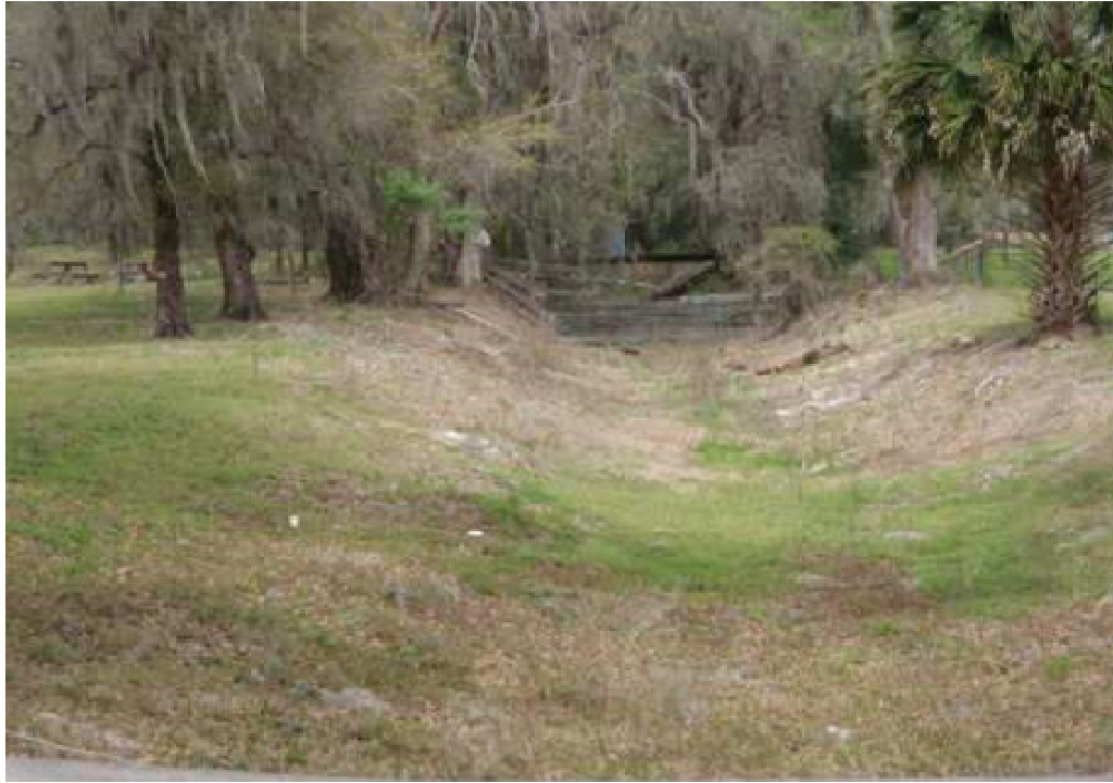
Figure 2: Dade City Canal in Florida is a man-made, mostly dry conveyance for flood control. Dade City Canal is not currently a water of the United States but would likely be deemed a “tributary” under the Rule. Fla. Stormwater Ass’n Comments 10, ID-7965 (JA__).
