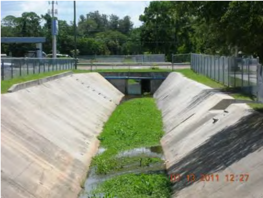
Figure 6: Ditch #5 in Pinellas County, Florida, is a manmade stormwater conveyance that discharges through a wetland into a navigable creek. It is already regulated as a point source. Under the Rule, it will be additionally regulated as a “water of the United States.” Fla. Stormwater Ass’n Comments 13 (JA__).
